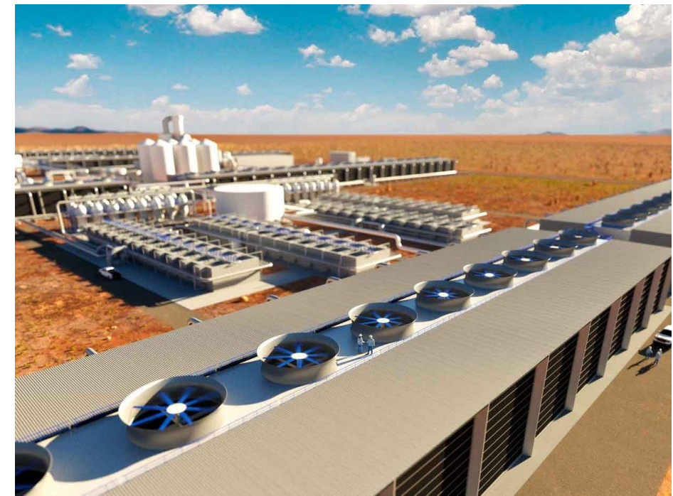
Carbon Engineering Direct Air Capture Plant (artist's image) – 1 Million tonnes/year CO 2 capture capacity
