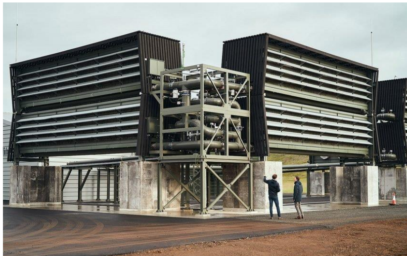
Climeworks' Orca Direct Air Capture Plant – 4000 tonnes/year CO 2 capture capacity
